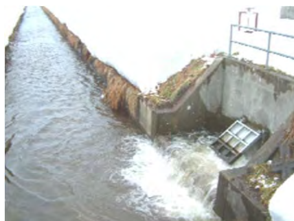
Fig.9 Pouring water for snow removal into the canal
