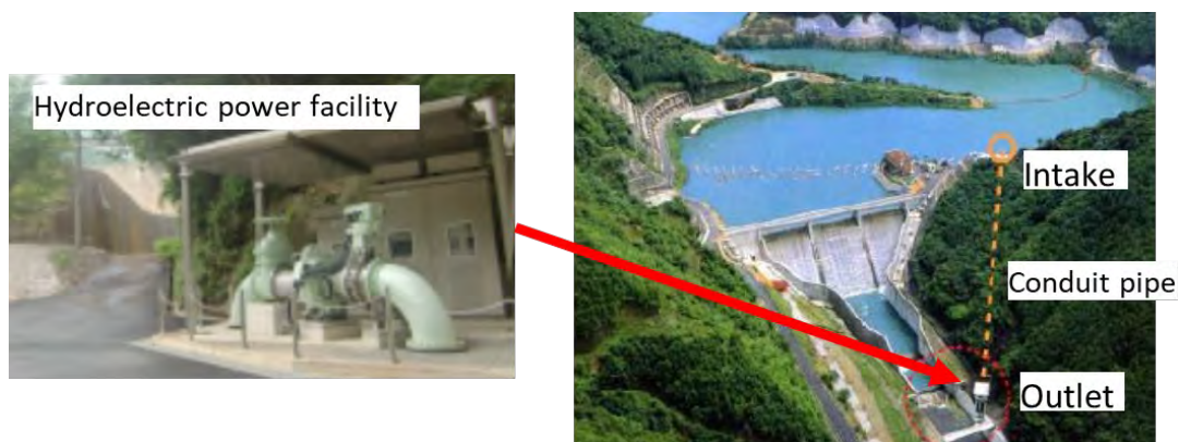
Fig.14 Nanki irrigation district (small-scale hydroelectric power generation at a dam)
