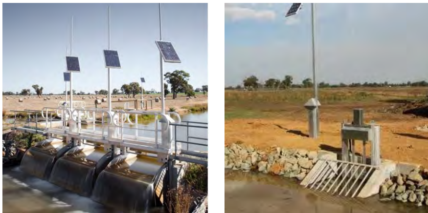
Figure 2 - GMID Modernised Infrastructure in 2020
